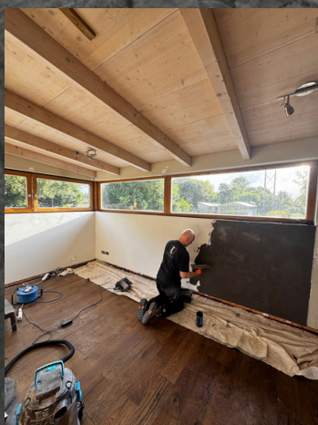
04 · SURFACE The system is covered and prepared for finishing.
