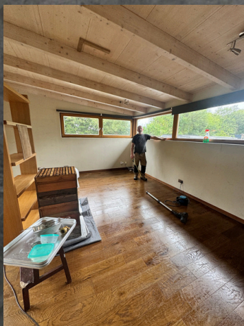
01 · HEATING ELEMENT The radiant heating material is positioned.
