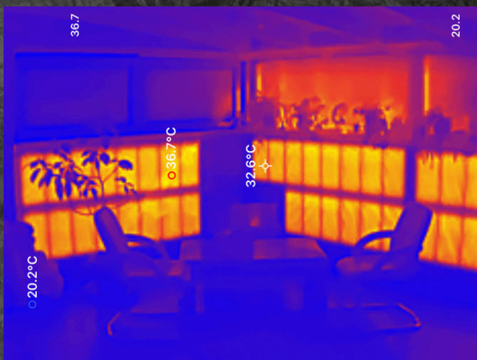
06 · THERMAL IMAGE The finished surface radiating heat.
